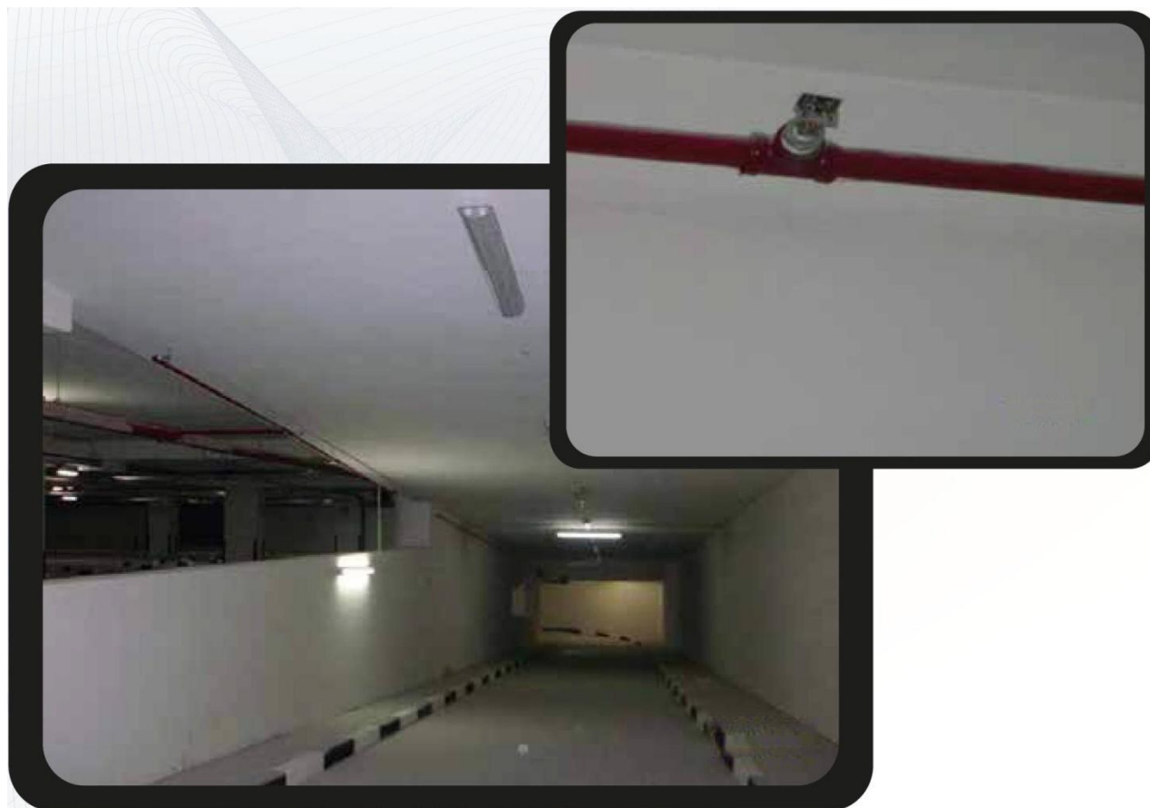
Installation of side wall Sprinkler
