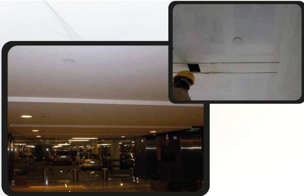
Installation of concealed Sprinkler
