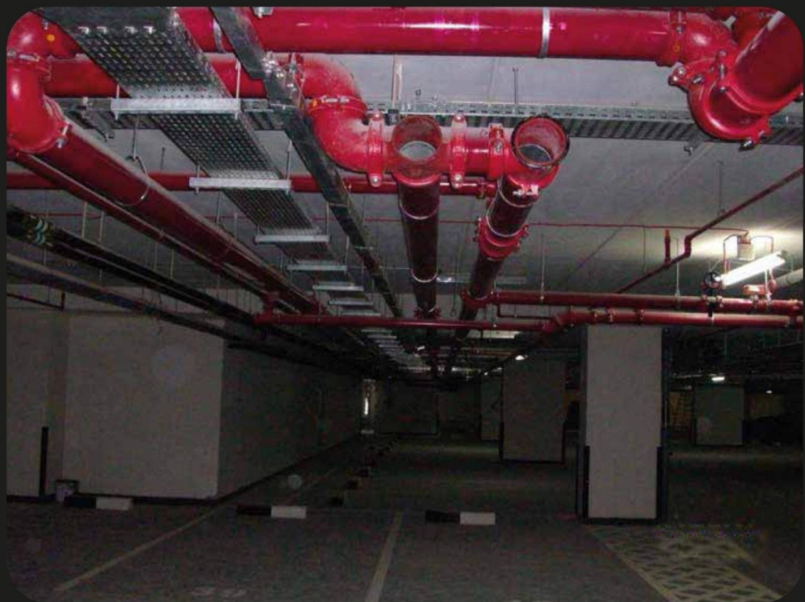
Header Pipes with Zone Control Valve
