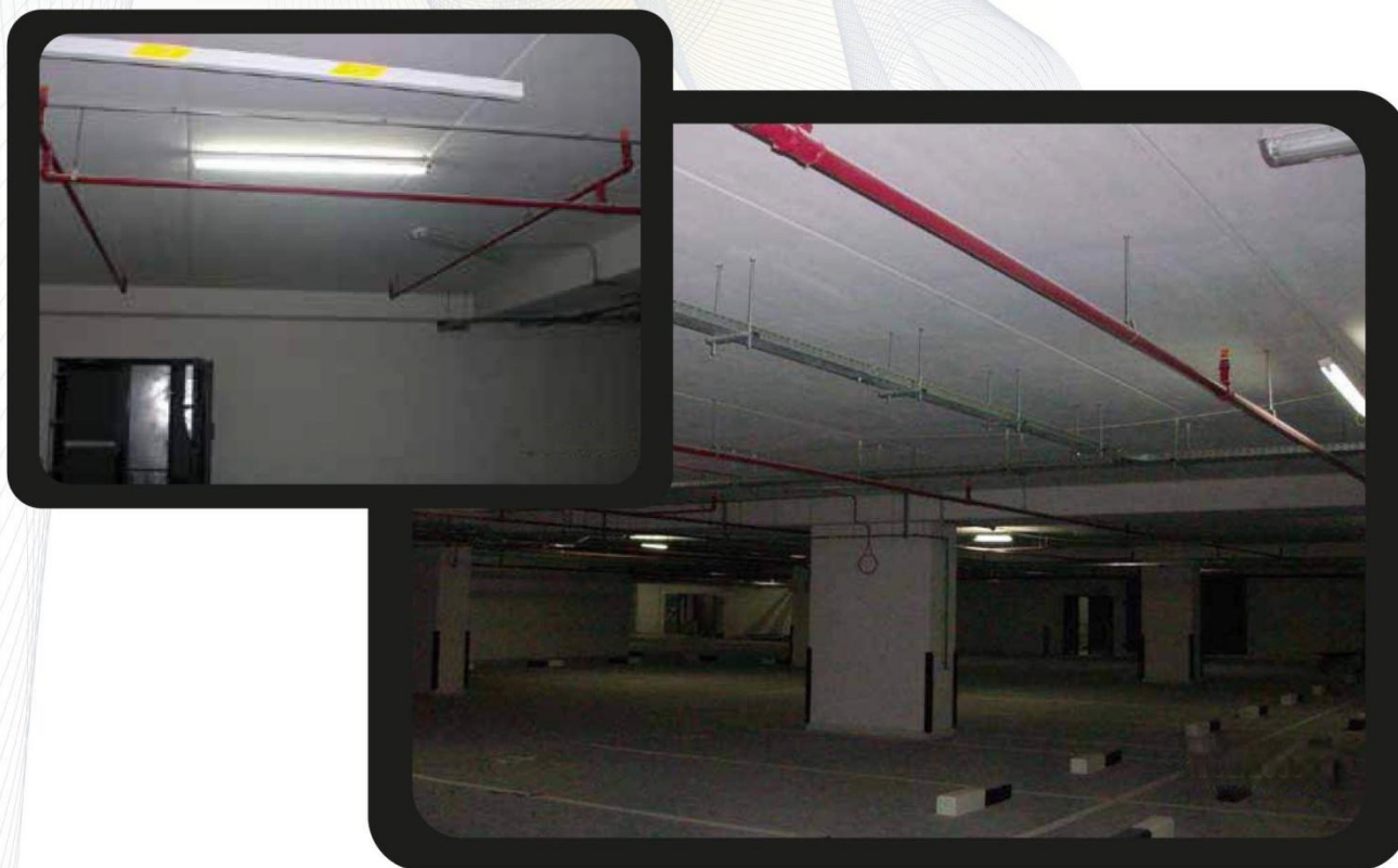
Installation of upright Sprinkler
